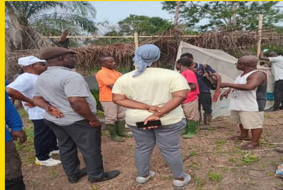
Site inspection of the 1.2mm culvert at Agyeibi-Asuogya-Bonkro feeder road
