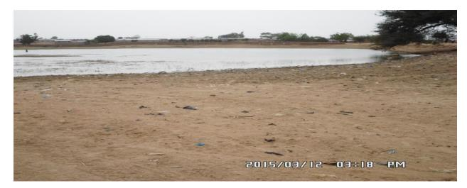
Photo 1: A silted dam at Abuss-Bawku
